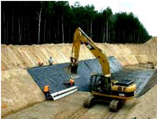
Technology of installation of anti-filtration polyethylene layer in the channel.
